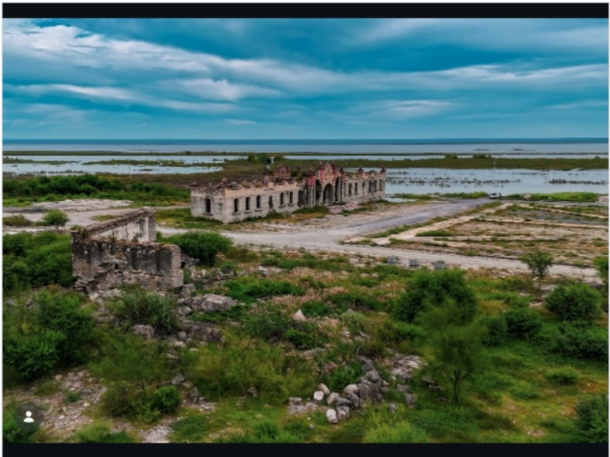
Fig. 7 With the reservoir's water level low, the local school can be seen in the background of the image. (Source: On instagram.com @tamaulipas_mexico, November 2024)
